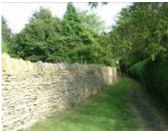
Boundary wall to footpath
